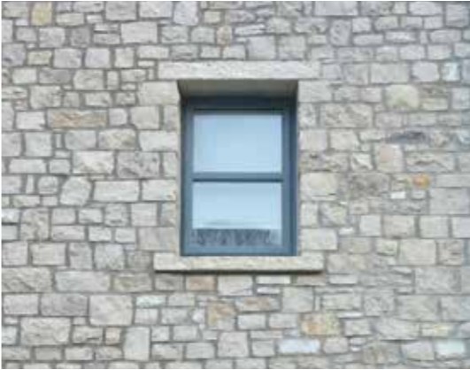
Baycliff limestone natural stone lintols and cills to any detail can be supplied to match the walling stone.
