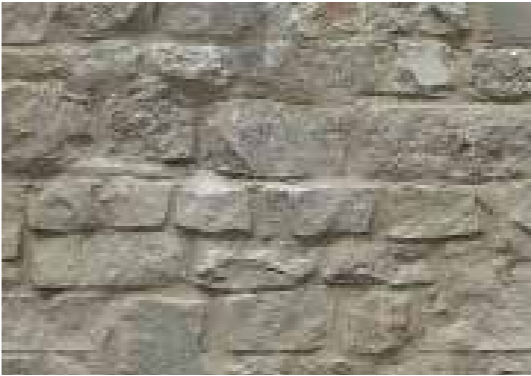
SQUARED RUBBLE WALLING
